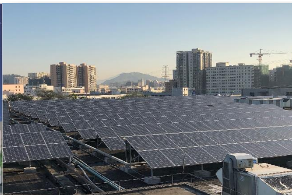
Rooftop PV System
